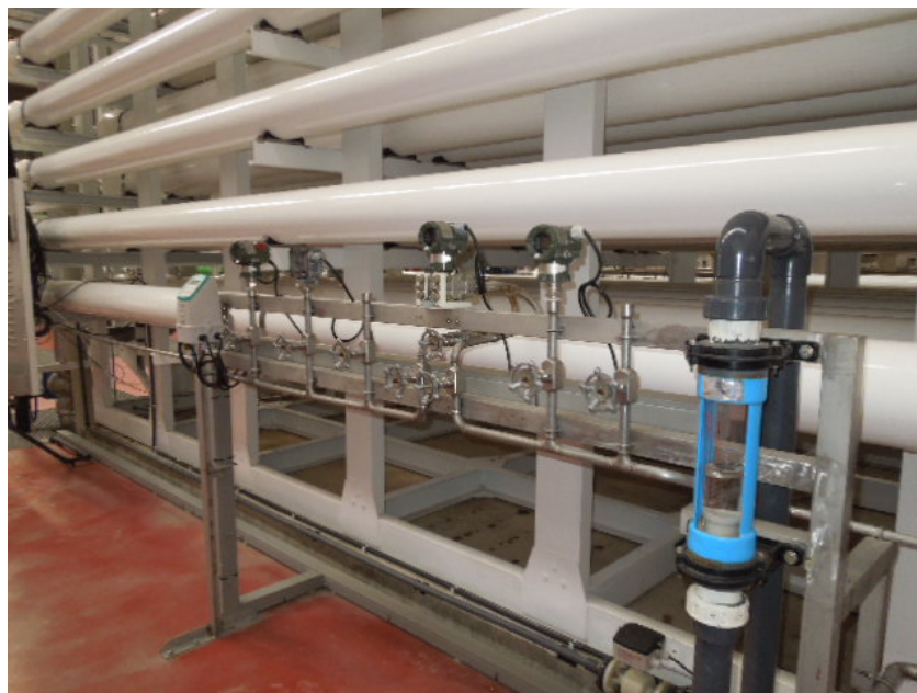
Figure 3: Pilot Test Pressure Vessel and Instrumentations
